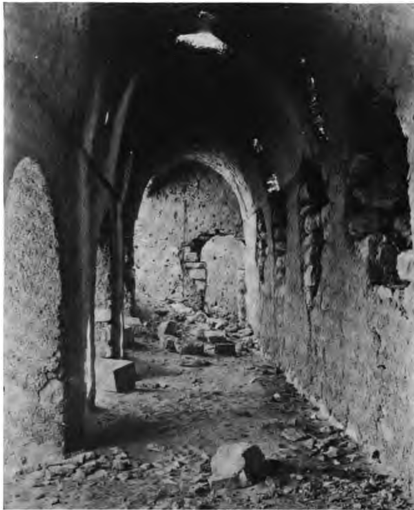
(b) The south aisle looking east.
